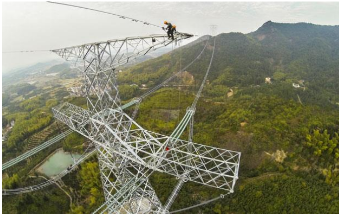
Big Grid: Electricians work on a 1,680-kilometer-long high-voltage DC transmission line that will move power from China's Xiluodu hydroelectric plant to Zhejiang province.
