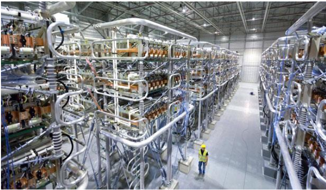
French Connection: A recently completed HVDC link between France and Spain doubles the amount of electricity that can be exchanged between the two countries. Converter stations like the one shown here sit at each end of the line, converting high-voltage AC to DC and DC back to AC.
