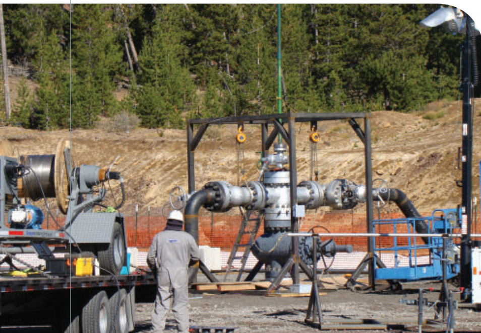
Drilling at AltaRock’s Newberry EGS Demonstration Project in Bend, Oregon. Credit: AltaRock.
