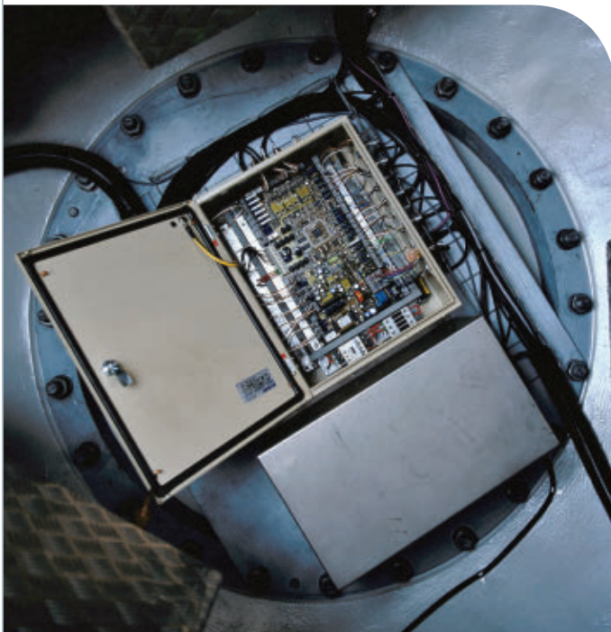
Figure 1. Wind turbine control panel.
