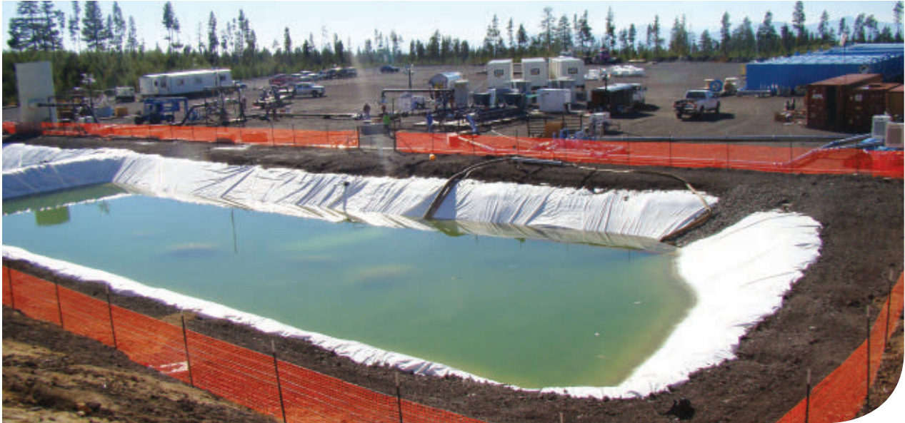
AltaRock’s Newberry EGS Demonstration site during stimulation. The pool holds fresh cold groundwater that was pumped down the 10,000 ft well during stimulation. Credit: AltaRock.
