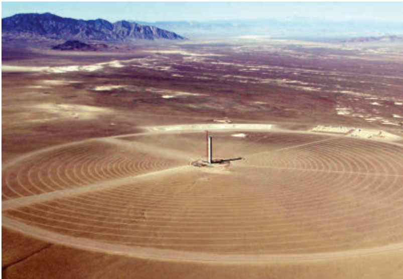
The 110-MW Crescent Dunes Project. Credit SolarReserve.
