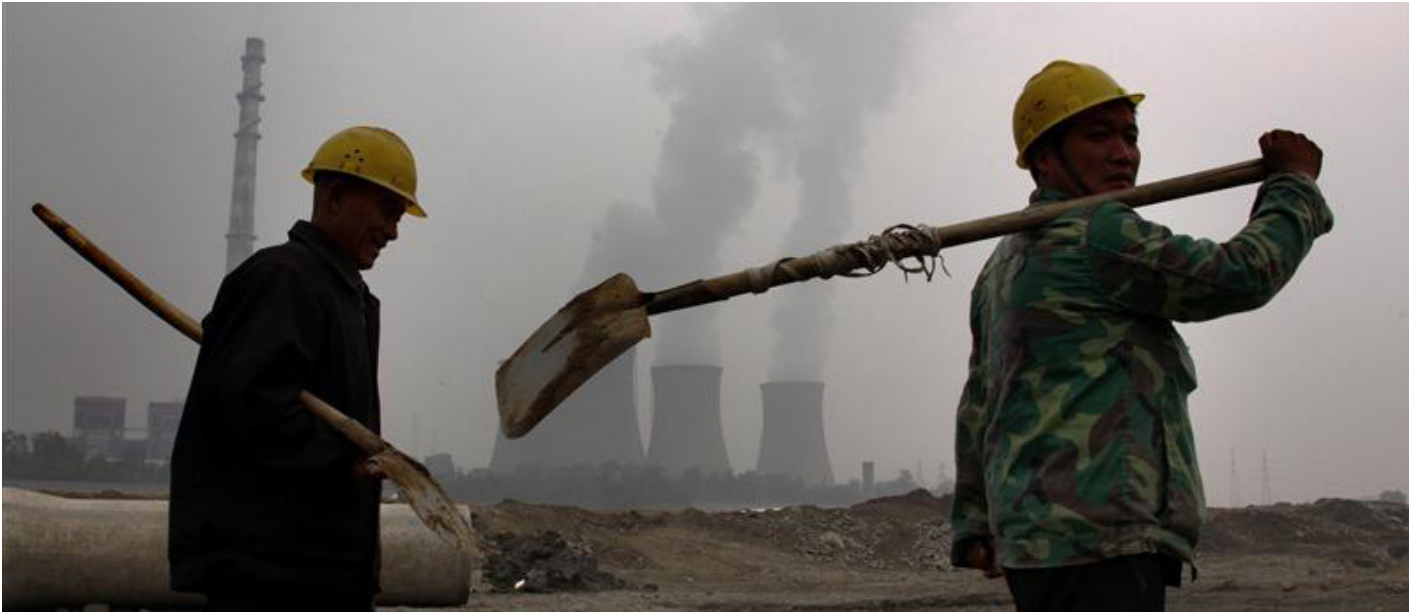
A coal-burning power station can be seen behind migrant workers as they carry their shovels on the construction site of a water canal being built in a dried-up river bed, located on the outskirts of Beijing on October 22, 2010. REUTERS/David Gray
