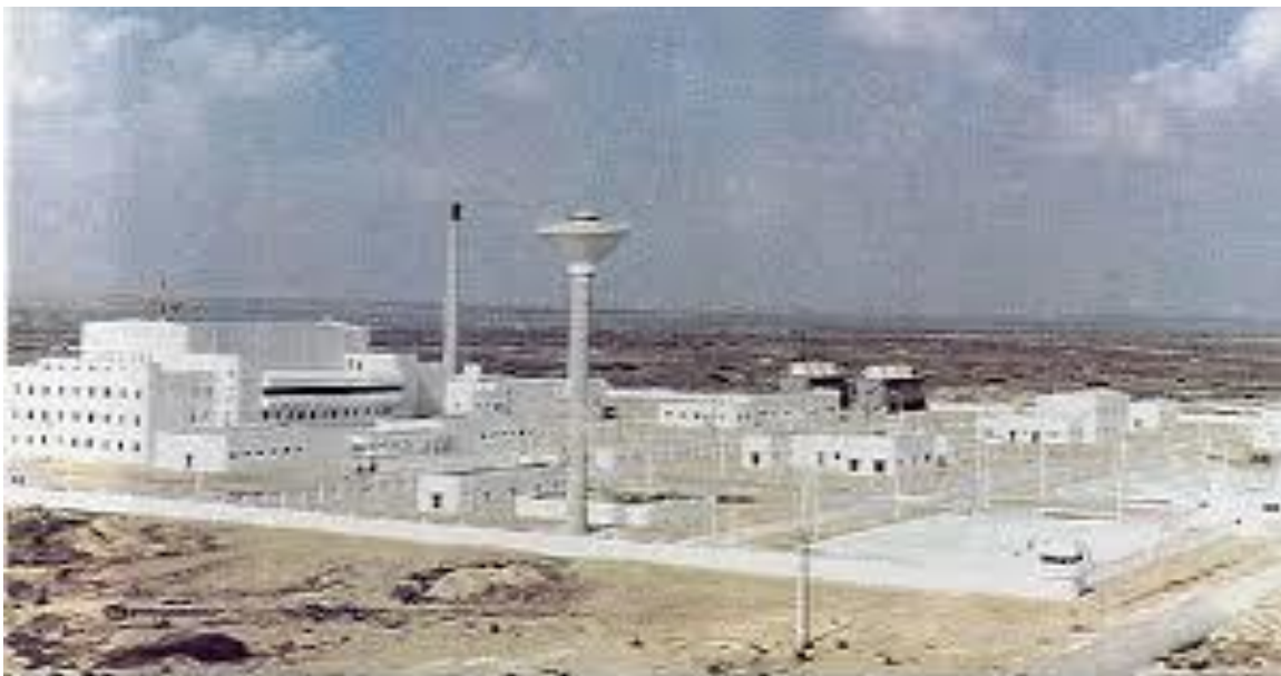
Figure 16- Birine nuclear research site. 25 Source: International Atomic Energy Agency
