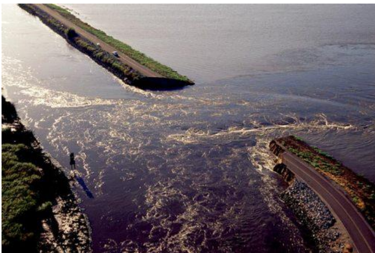
Figure 15. Image taken on June 3 rd , 2004, of the Upper Jones Tract levee break. From Romick 2009
