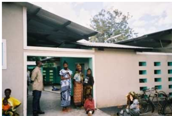
This hospital in Tanzania receives its electricity from solar panels
