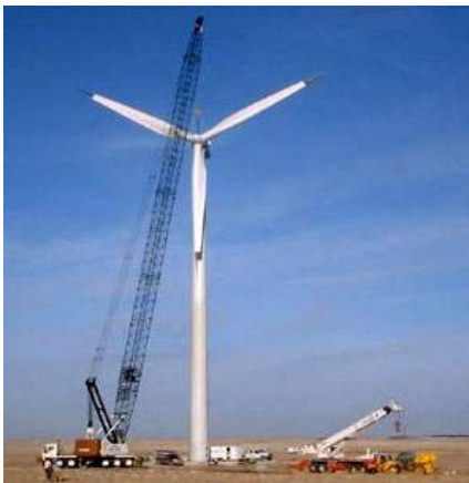
Fig 11, the construction of the Rosebud Sioux 750 Kilowatt turbine. Source: http://www.wapa.gov/ES/pubs/esb/2003/03oct/esb102.htm
