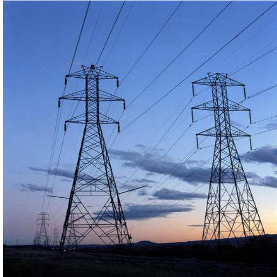
Fig 13, a small part of the vast U.S. transmission grid. Source: www.eere.energy.gov .
