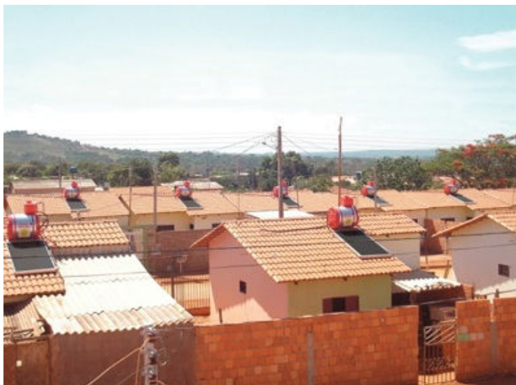
FIGURE 16: SOLAR WATER HEATING SYSTEMS ON BRAZILIAN HOUSES
