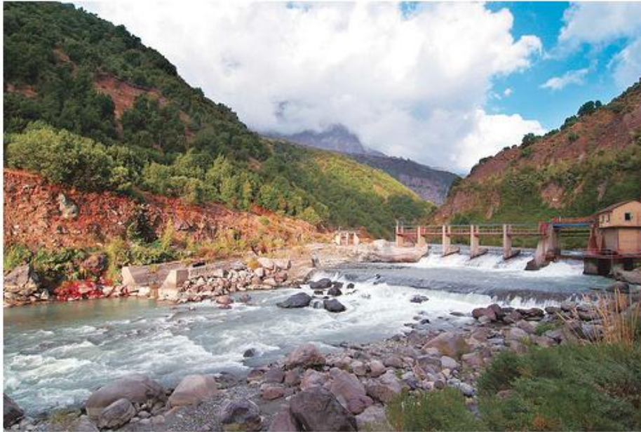
Figure 14: Coya and Pangal hydropower plant
