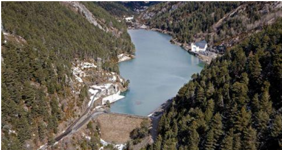
Figure 47: Lasarra Hydropower Station in Aragón, Spain
