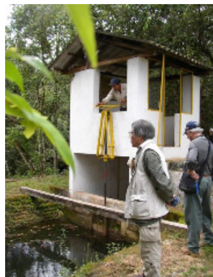
Figure 21: Micro-hydropower plant in Gaviotas, Colombia
