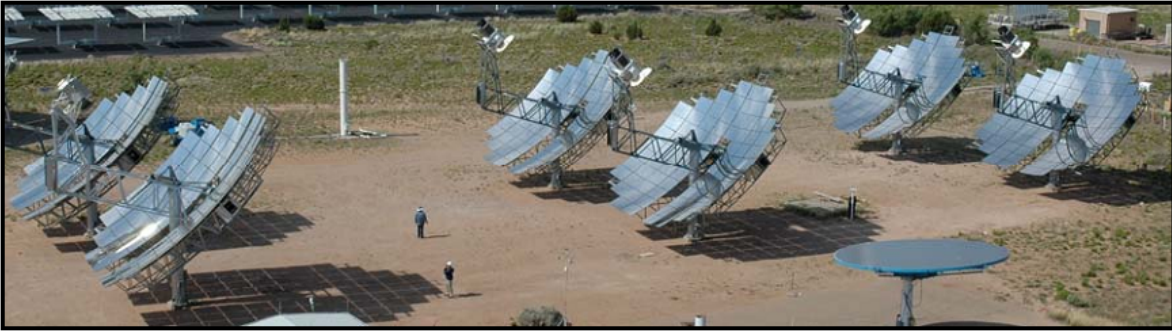
Figure 14: Prototype 150 kW dish/Stirling Power Plant at Sandia National Laboratory
