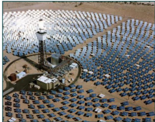
Figure 5: Aerial of Solar Two in the Mojave Desert in California
