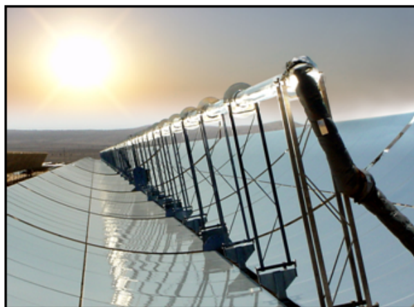
Figure 11: Solar Parabolic Troughs
