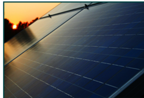
Figure 7: Residential Photovoltaic Panels
