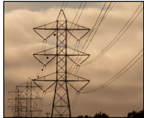
Figure 22: High Capacity Transmission Lines in California
