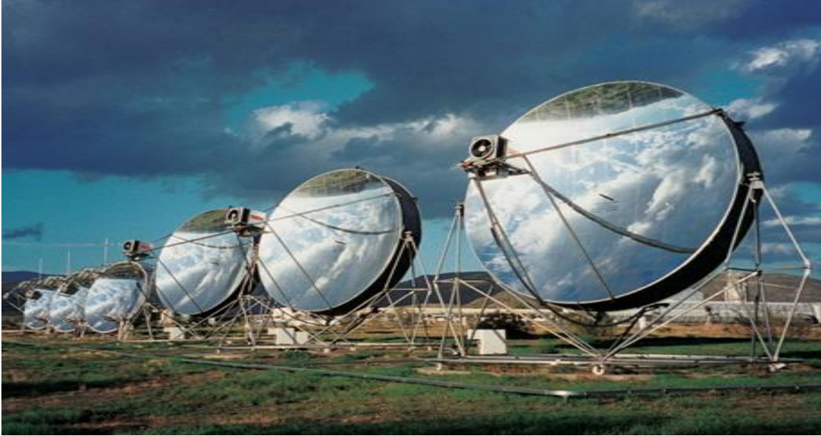
Figure 11: Stirling dish power plant
