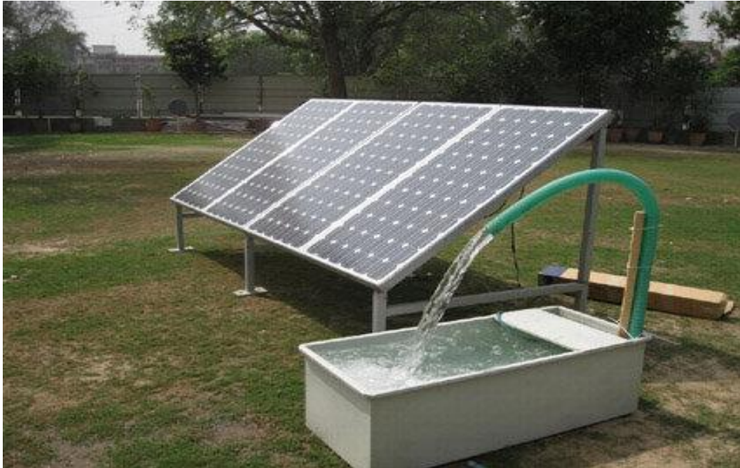
Figure 18: Application of solar water pumping system Source: (Dr. Solar)
