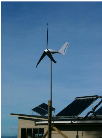
Figure 9: A roof-mounted wind turbine
