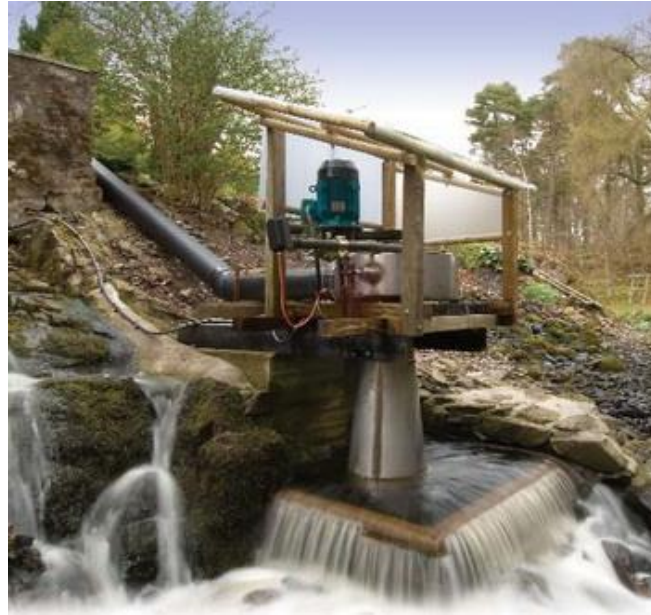
Figure 13: A small hydropower station
