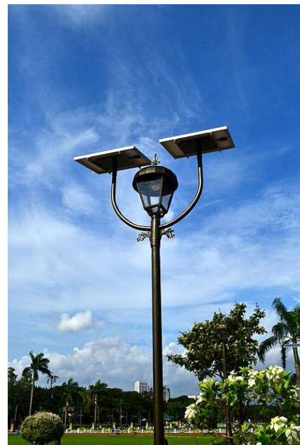
Figure 5: A LED light run by solar panels
