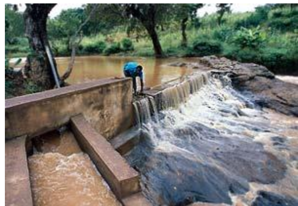
Figure 15: A small dam was built to divert water
