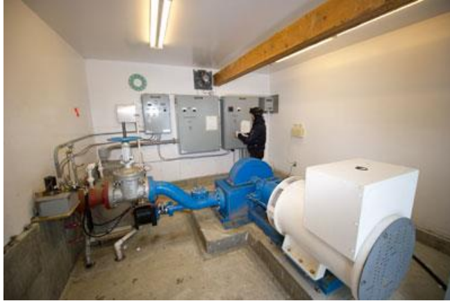
Figure 14: The peripherals of a small-scale hydropower system
