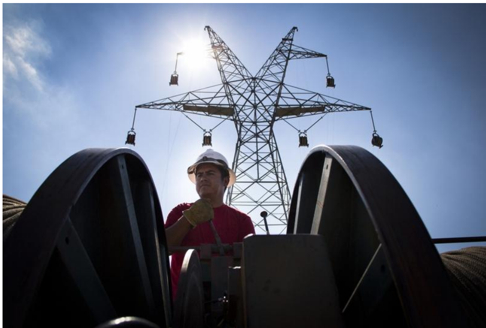
Figure 11: Construction of Wind Energy Transmission Power Lines Near Sweetwater, Texas
