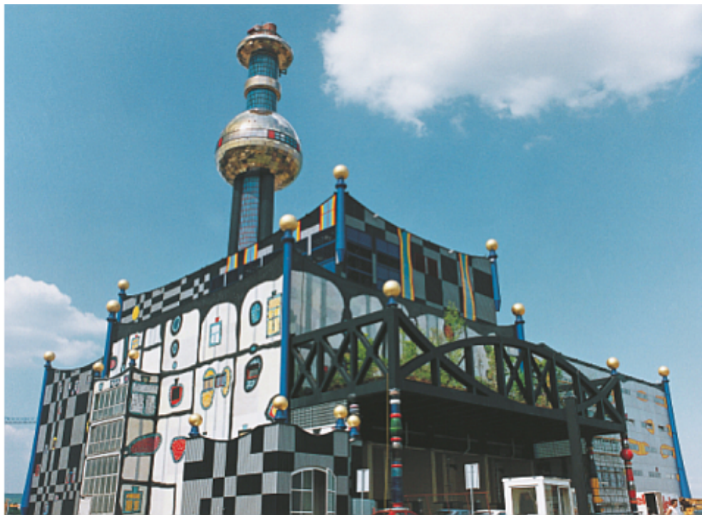
Figure 22: The Spittelau waste-to-energy plant in Vienna, which now generates heat 23
