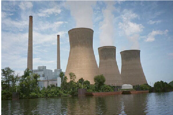
Figure 4: Power Plant on the Ohio River
