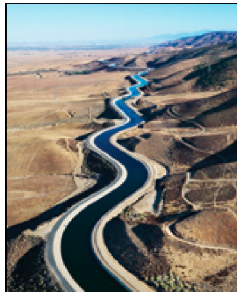
Figure 3: The California Aqueduct
