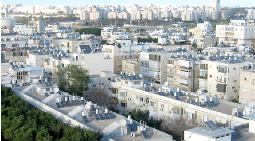
Figure 28: Rooftop Solar Water Heaters in Israel
