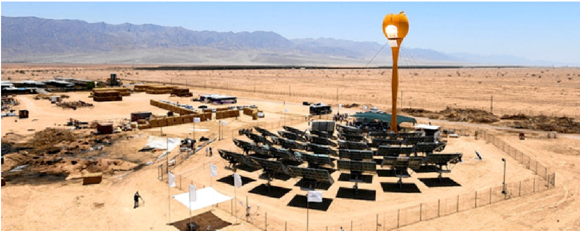
Figure 29: Arava Power Company's 4.9-Megawatt Solar Tower Facility
